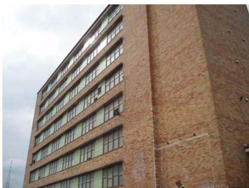
Above: Sturt House will be demolished later this year.
